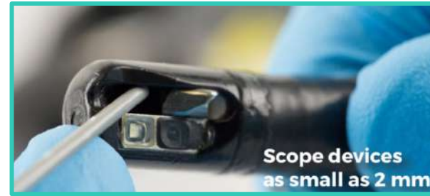
Insert behind the elevator riser
